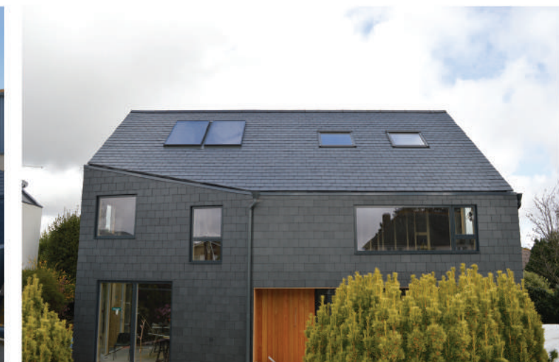
Prestige roofing contractors demonstrating Merayo's versatility
