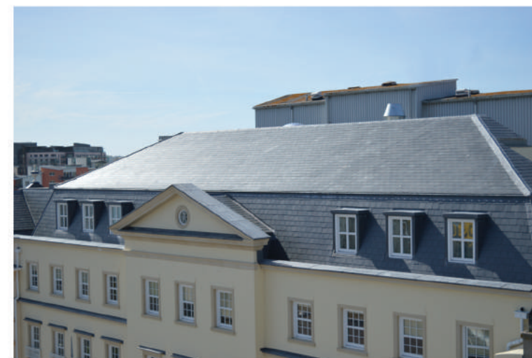
Double award winning heritage project in Jersey
